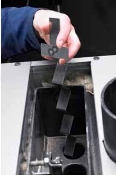
Remove all turbulators.
